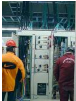
Aurul – Gold extraction plant
